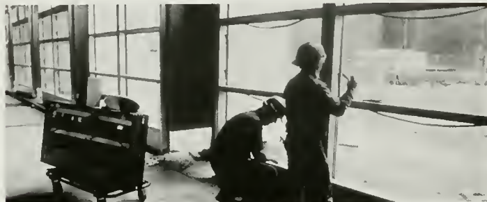
Saflex® being installed in Eagleton Federal Building, St. Louis
